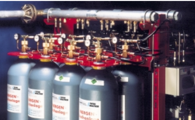
A space-saving INERGEN® 200bar cylinder battery
